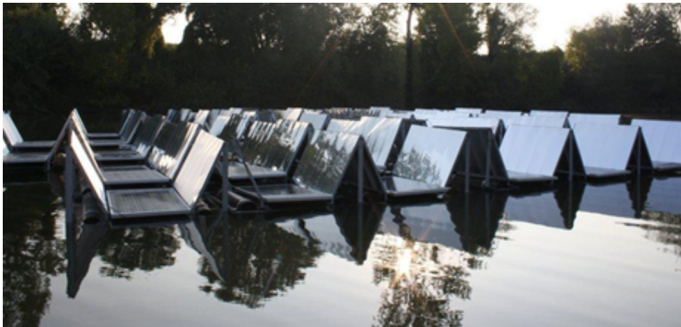
Figure 1.9: Floating PV with reflector "V-trough" solution [7]
